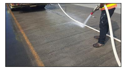
13. Washing is to remove any excess material sitting on the surface. Washing should be done with clean, clear water. Washing should continue until there is no "white foaming" occurring, which is evidence of the presence of the material.
