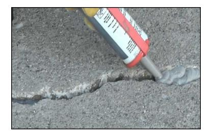
ACR PolyMembrane Flashing application rates will vary, but under most conditions when applying 30 mils dry thickness, it will require 2.3 gallons per 100 square feet. (8.7 liters per 9.3 square meters) or 217 square feet per 5 gallon bucket. At 40 mils dry thickness, it will require 3.1 gallons per 100 square feet (11.7 liters per 9.3 square meters) or 163 square feet per 5 gallon bucket.
