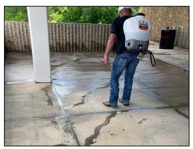
16. After spraying allow all surfaces to dry to the touch. Once all surfaces are dry to the touch, beginning washing off excess materials from the surface. Washing should continue until there is no "light white foaming" occurring, which is evidence of the presence of the materials.
