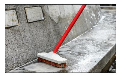
ACR Concrete Masonry Cleaner - Use this product to remove dirt and environmental debris. This product is sprayed on the surface and in most cases will require some agitation. Once the dirt and debris has been removed rinse with water. Coverage rate for this product will vary depending surface condition, but when used as directed the coverage rate is approximately 400-500 square feet per gallon. This product should be used at full strength.
