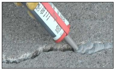
ACR PolyMembrane Flashing application rates will vary, but under most conditions when applying **30 mils** dry thickness, it will require 2.3 gallons per 100 square feet. (8.7 liters per 9.3 square meters) or 217 square feet per 5 gallon bucket. At **40 mils dry thickness**, it will require 3.1 gallons per 100 square feet (11.7 liters per 9.3 square meters) or 163 square feet per 5 gallon bucket.
